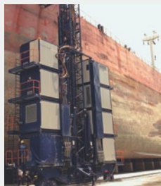
Automated hull blasting and coating...
